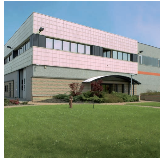
Production site Siziano (PV)
